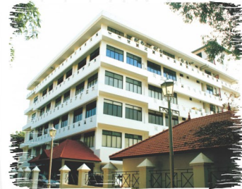
Seaview Support Systems Building, Technopark, Trivandrum
